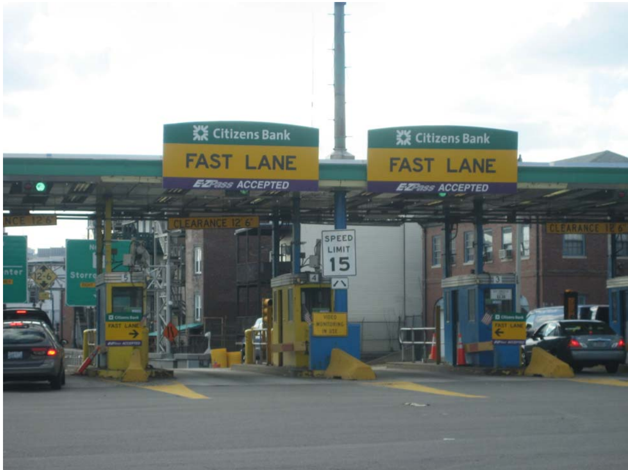
Sumner Tunnel entrance.
